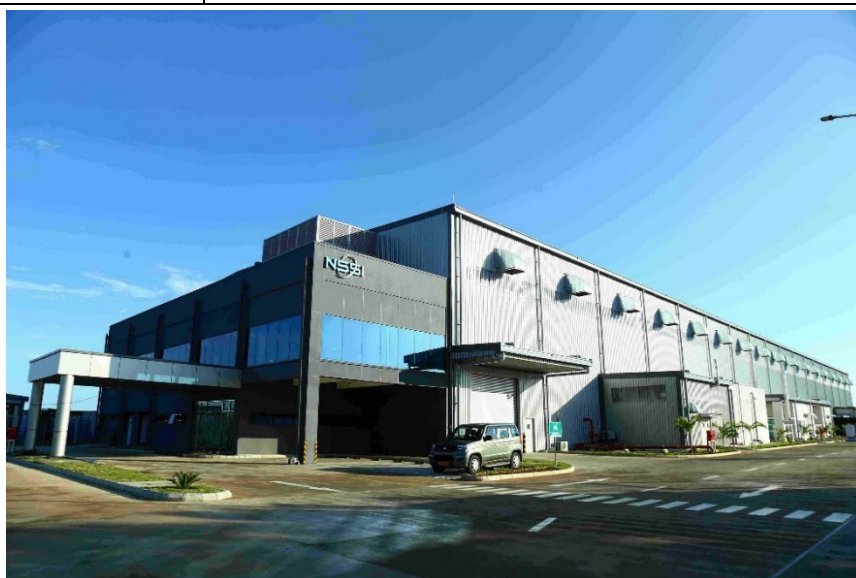
Appearance of Factory No. 2
