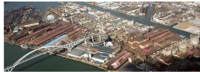
Nakayama Steel Works (Osaka)
